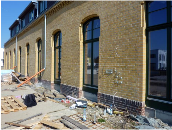
Figure 9. Tested historical fair-faced masonry façade in Leipzig, Germany.
